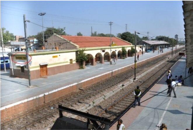
Railway Station Shikohabad
